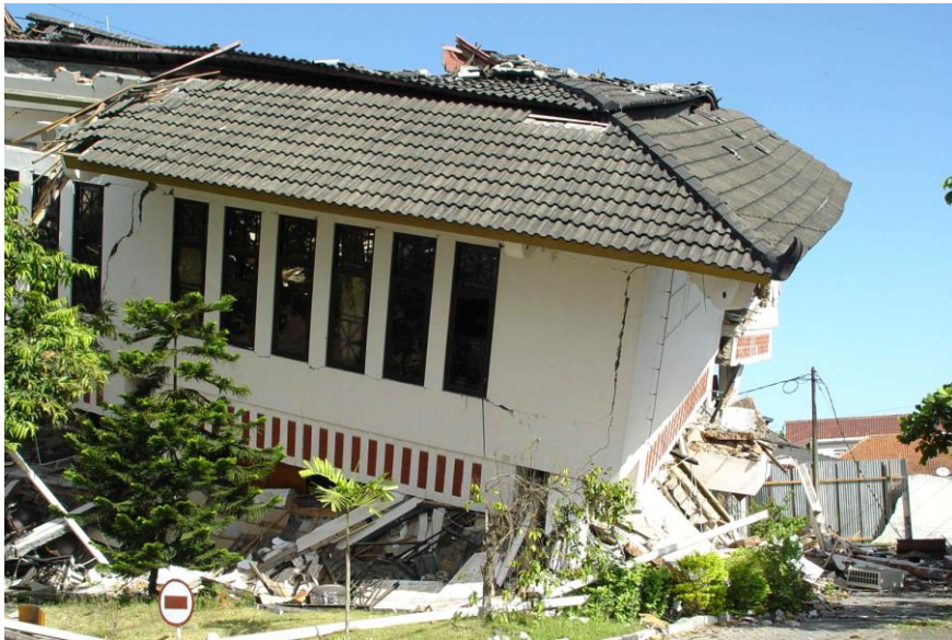
Figure 2-3 Yogyakarta Earthquake in 2006
