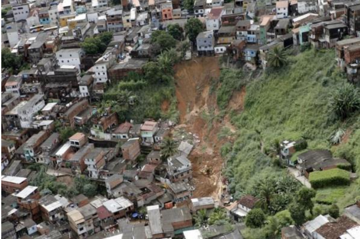
Figure 4-2 Landslide from heavy rainfall, Brazil
