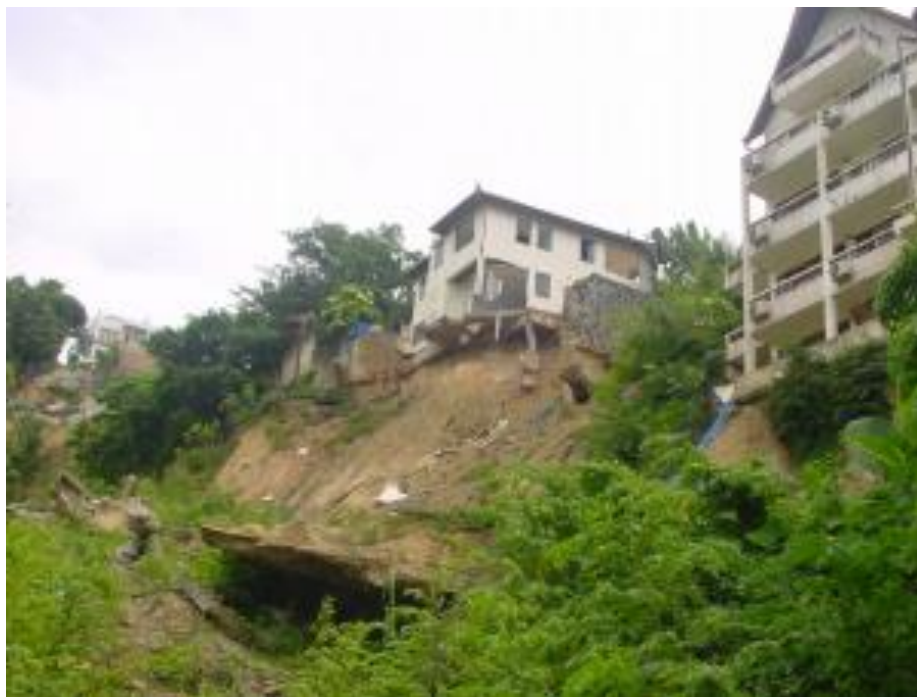
Figure 4-1 Na Nai roadside landslide on October 25, 2007
