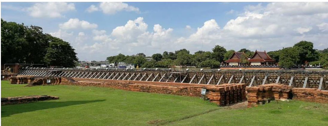
Figure 6-3 Floodwall along the Chao Phraya River at Wat Chaiwatthanaram
