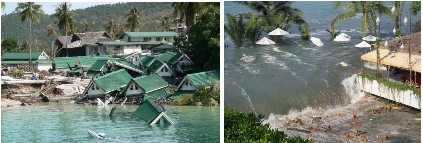
Figure 8-6 Damage of Tsunami on Phi Phi Island, Krabi province, Thailand in 2004
