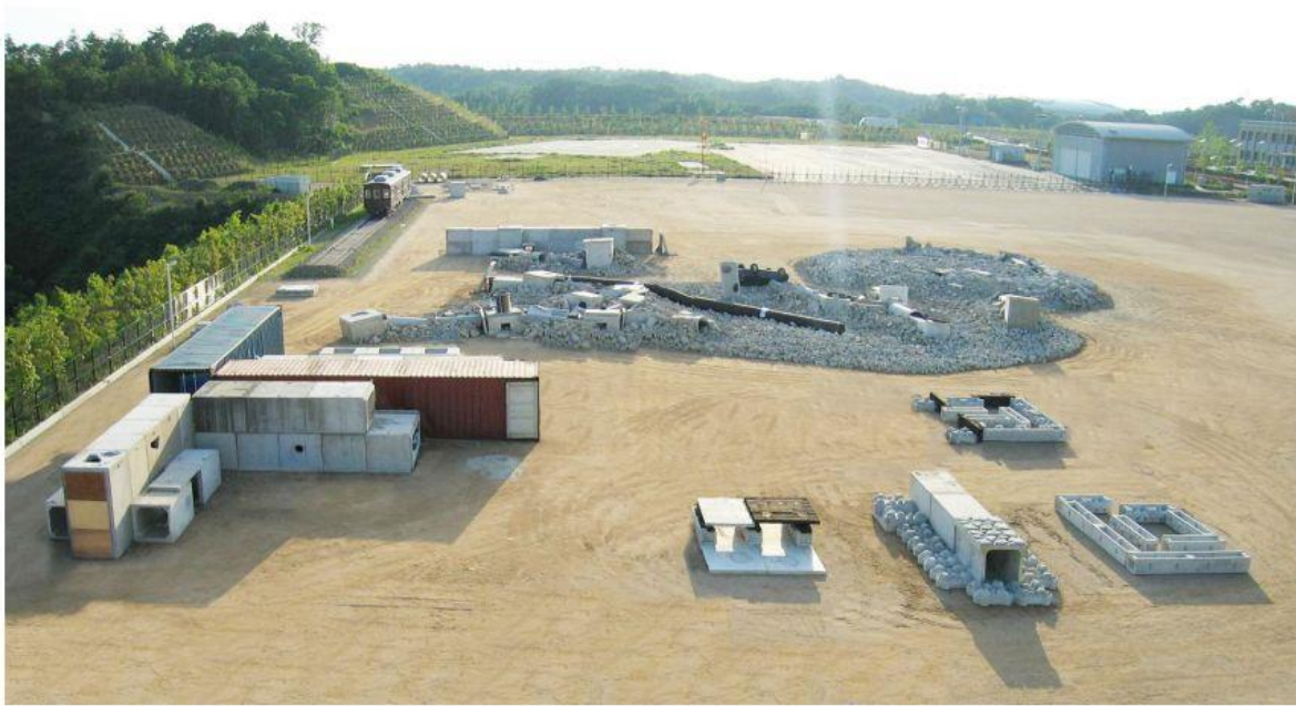
Figure 4-7 Hyogo US&R training facility
