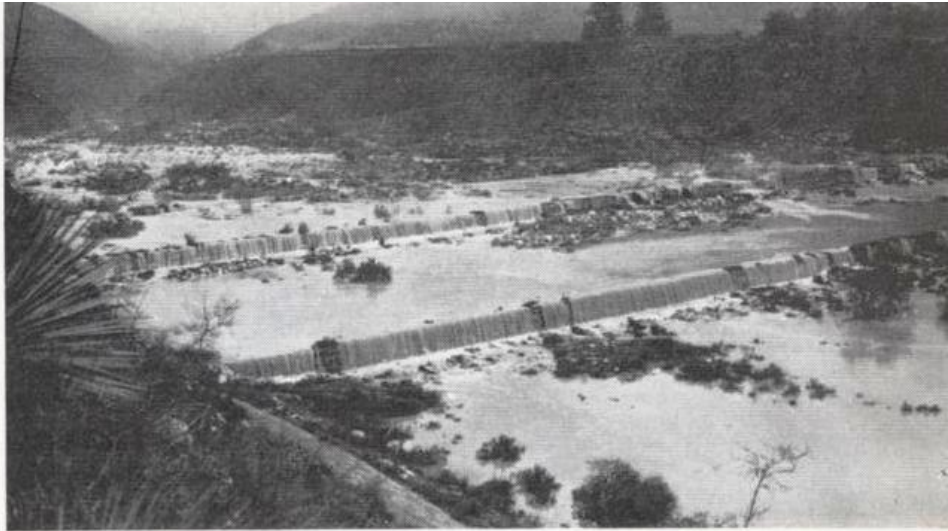
Fig. 13.3 Channel spreading with rock-and-wire check dams in Cucamonga Creek near Upland, California (courtesy D. C. Muckel).
