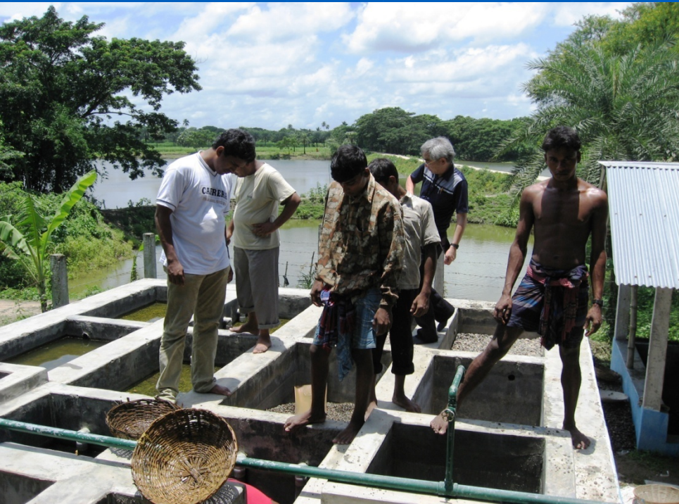
Washing of gravel and sand in the filter
