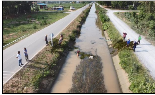
Fig. 5. Wheelbarrow rake set. For canals with a bottom width of 1.0 to 2.0 meters.
