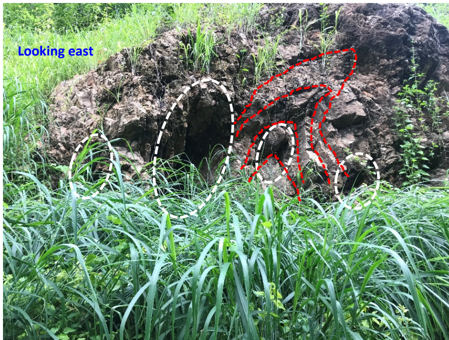
Fig. 1. Rock exposures at Huai Khun Mi, showing opened joint, fracture, and cavity (white), associated with fold structure (red) as channels that water outflowing from reservoir.
