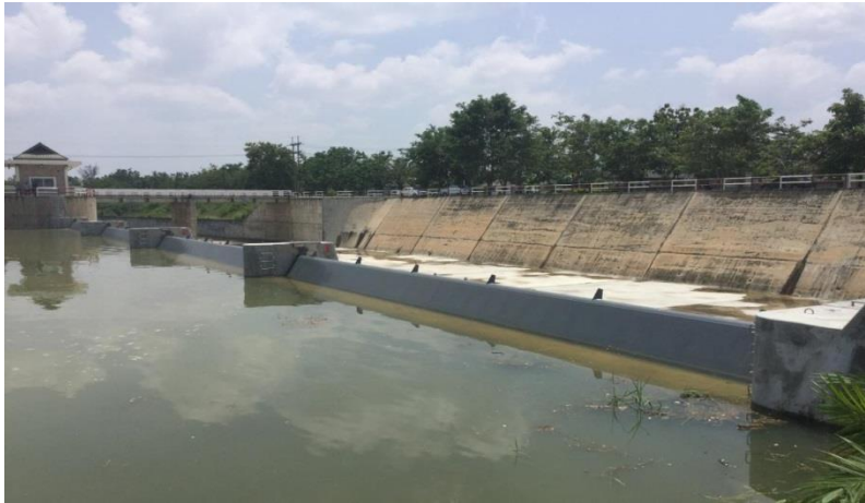
Prasae Reservoir Install a Type III-A folding dam to start collecting water to help prevent flooding at the bottom of the reservoir.
