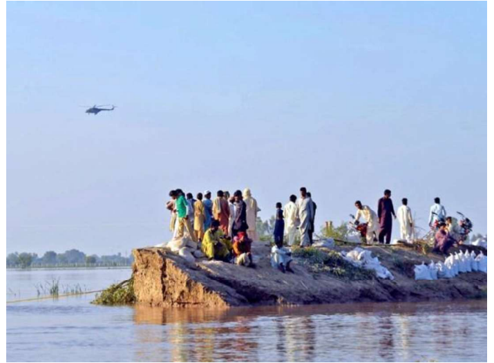
Breached flood bund of Chenab River
